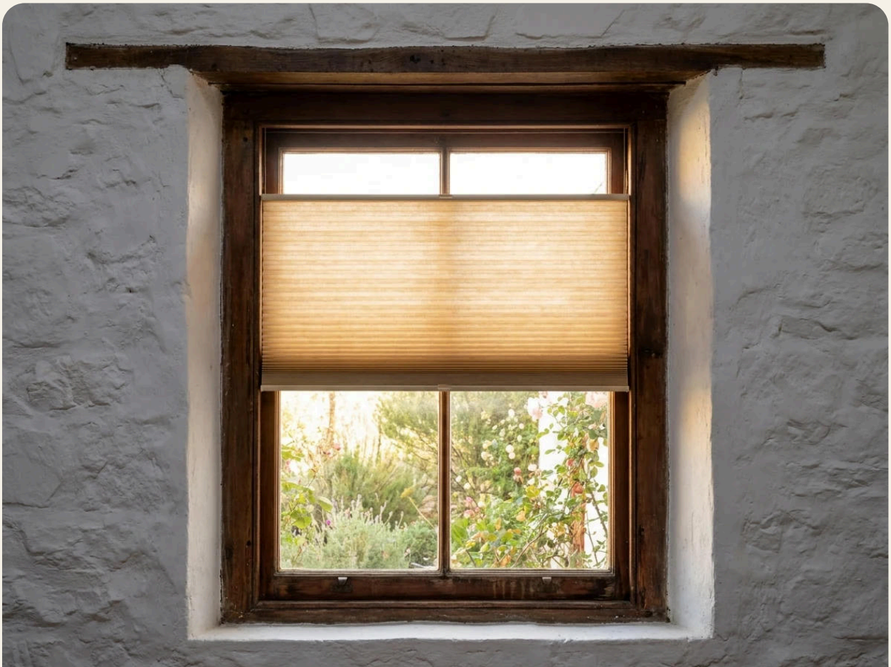
Stanford — inside the reveal of a village cottage window, where the honeycomb is working against a cold night rather than a bright sea.
